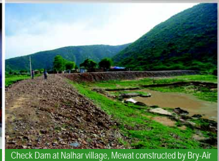
Check Dam at Nalhar village, Mewat constructed by Bry-Air
